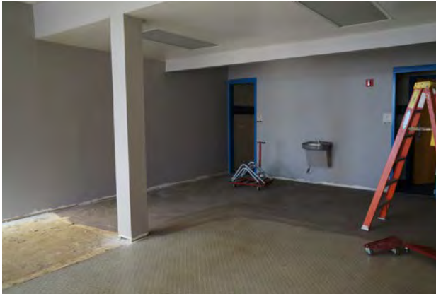
11 Child Care (under construction)
