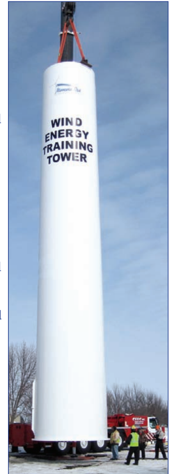
Canby Wind Energy Training Tower
